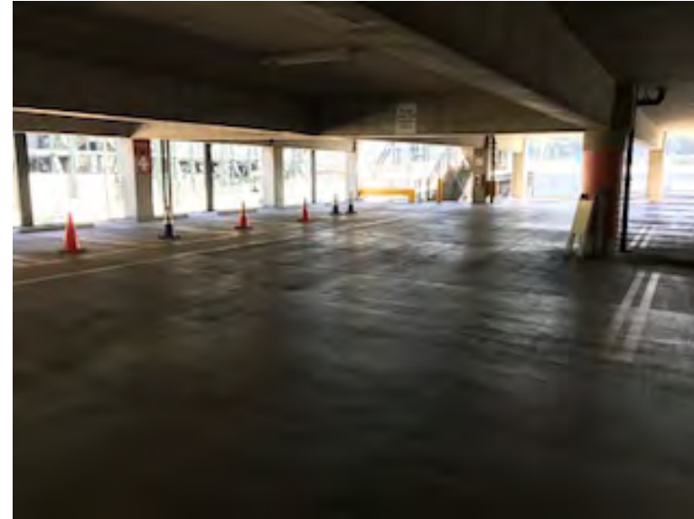
Level three looking north, showing good condition
