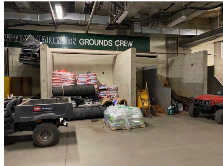
Groundskeeping space was observed to be well organized and clean
