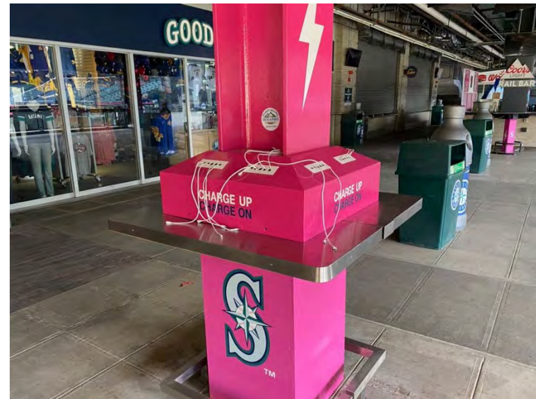
T-Mobile phone charger location at The Pen requires fans to stay with phone – consideration should be given to adding a secure, lockable phone charger station so fans can return to their viewing location or seats
