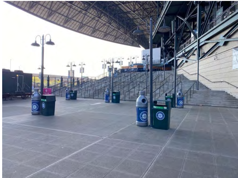
Center field gate location is in good condition and very clean
