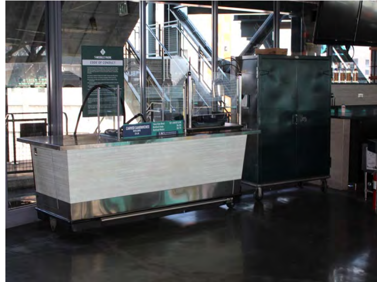
Concession area, this area was clean and in fair condition equipment looks dated
