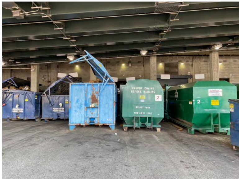
Loading dock with the dumpsters for trash and recycling is well maintained and clean - Operations is going to replace the asphalt and the rails in 2021 offseason
