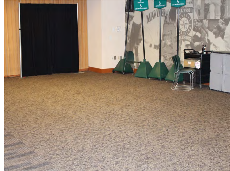
Ellis Pavilion carpeted floor in good condition
