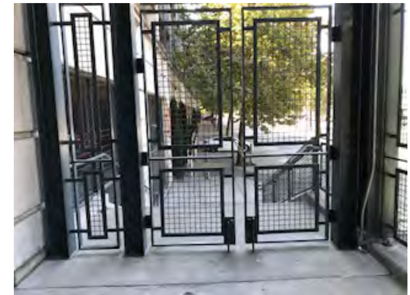
Exit doors looking west on level two in good condition
