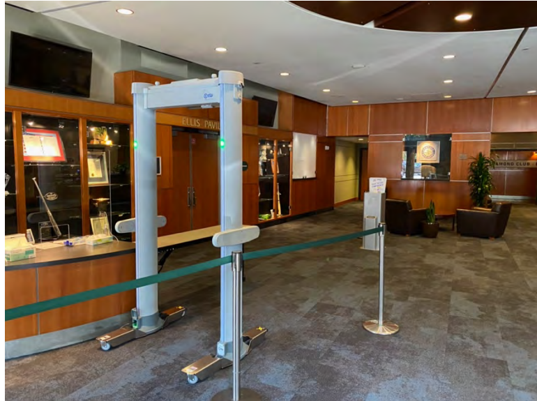
Third base entry was observed to be in good condition
