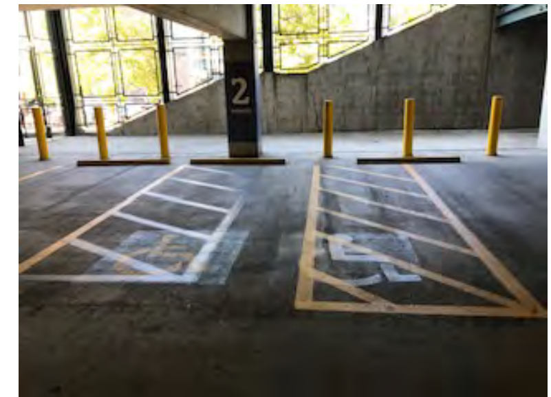
Just inside the main entrance paint on the surface is confusing and should probably be redone
