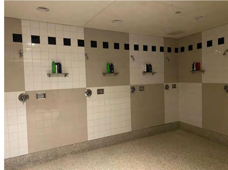
Wet area was observed to be well maintained
