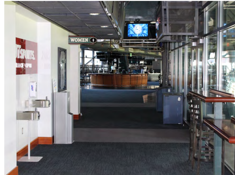
Corridor carpet is clean and in good condition
