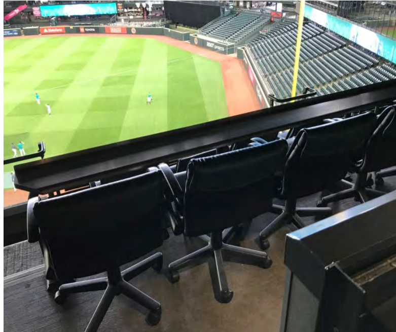
Exterior of suite in good condition, some chairs showing wear
