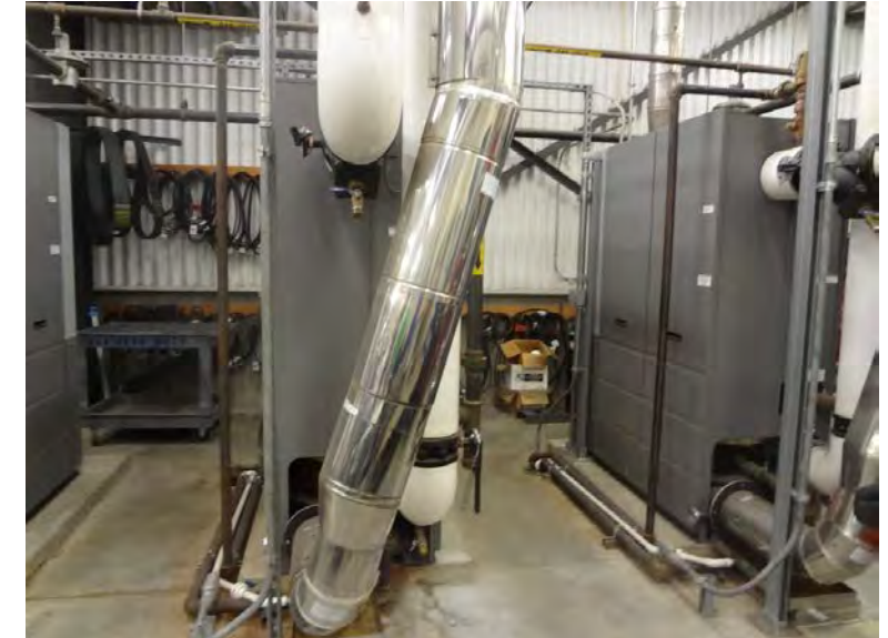
Central plant is clean but somewhat cluttered
