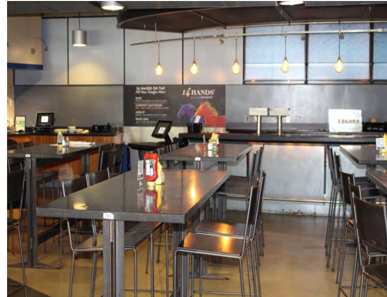
Interior of Hit It Here Cafe has tired finishes
