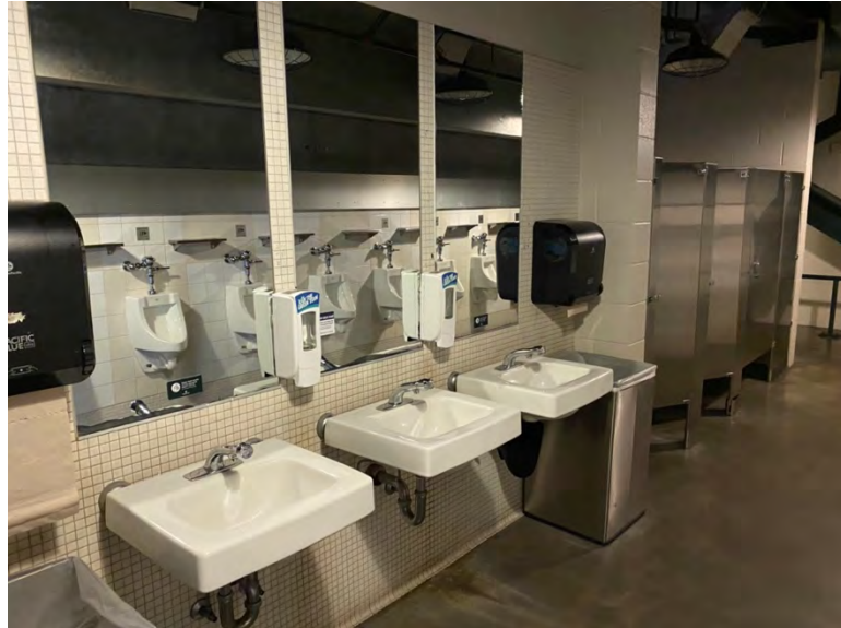
These sinks should be replaced with a slab sink at time of renovation
