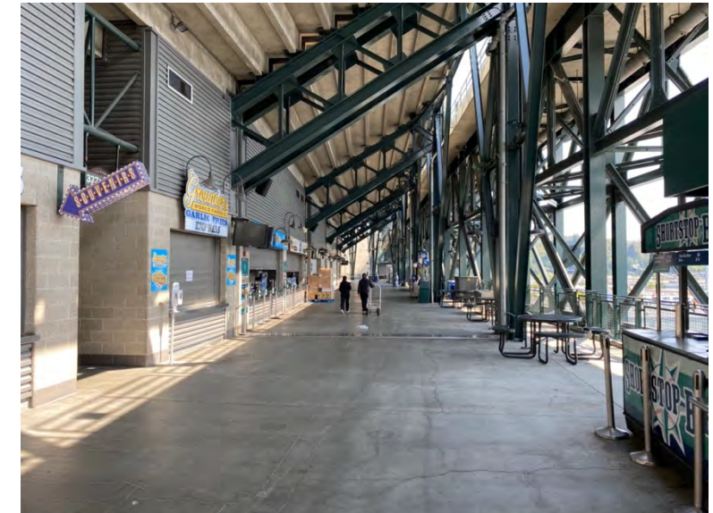
Upper Concourse outside section 331 has been well-maintained
