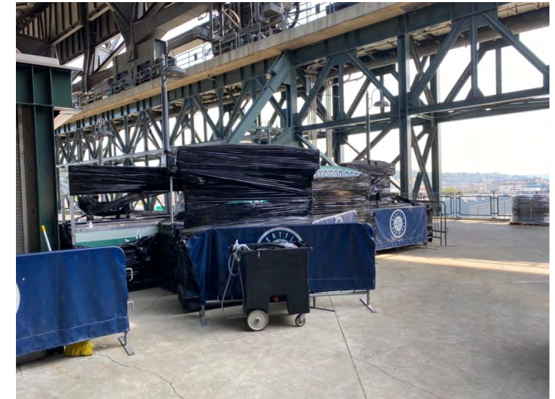
Concession portable storage on the concourse outside Section 314 is visible to the fans – recommend placing windscreen to block the view of fans into the “boneyard”
