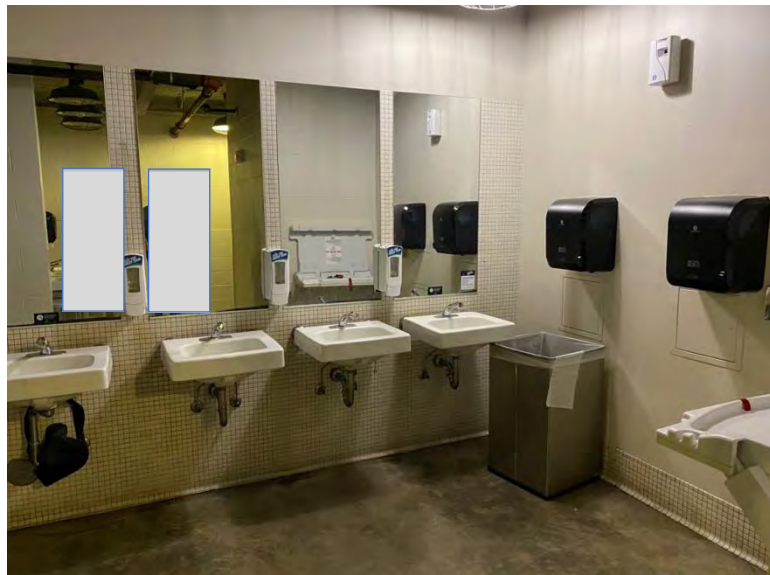
Men's restroom outside Section 112/114 is in good condition as the finishes are original and are likely due for an upgrade in the next couple of years
