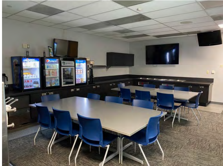
Player dining area was observed to be well maintained
