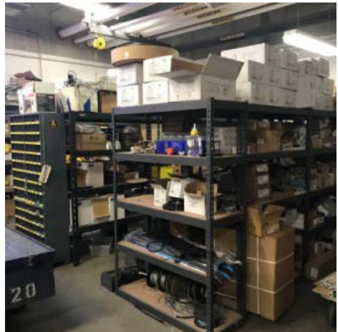
Unsupported Storage Racking in Maintenance Area
