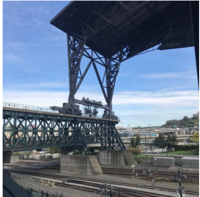
Roof Support Truss and Steel Structure
