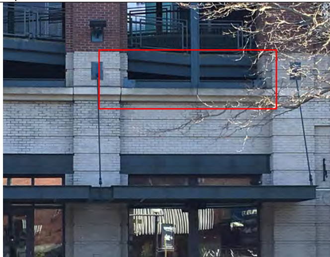
Saddle flashing installed at both ends of beam.
