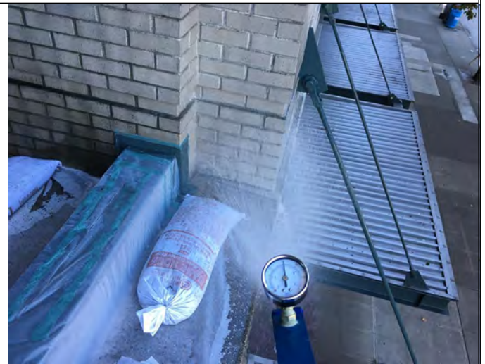
Isolation water test procedure.
