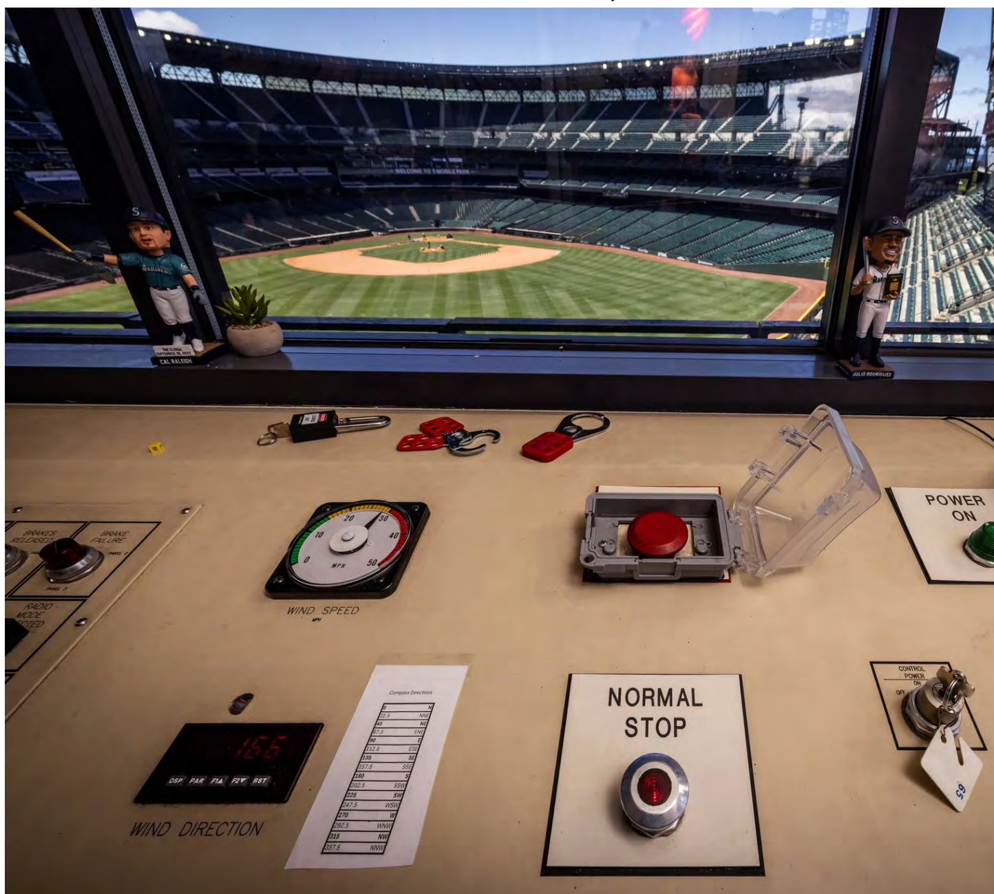
Two stop buttons for T-Mobile Park's retractable roof, including the larger red "emergency" one, are in the control room overlooking the baseball field and seats. (Ken Lambert / The Seattle Times)
