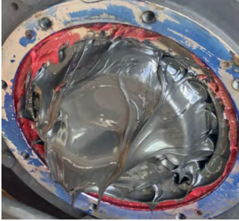
Over-worn, overloaded bearing. Dark grey grease. G5 wear
